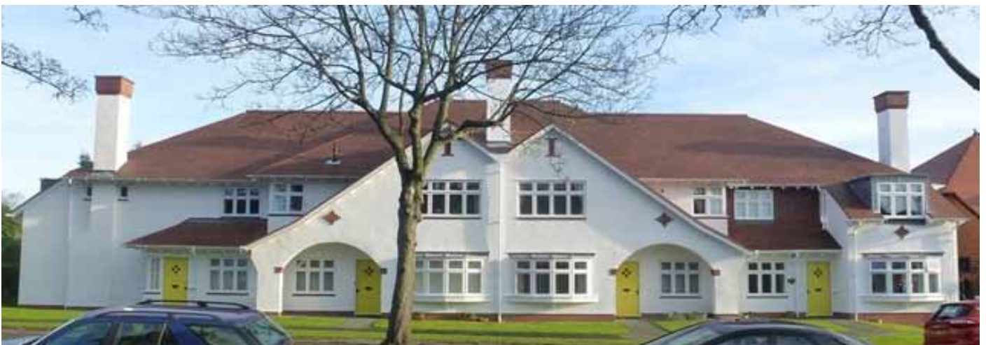
Cottages on Central Road © Rory Walsh
