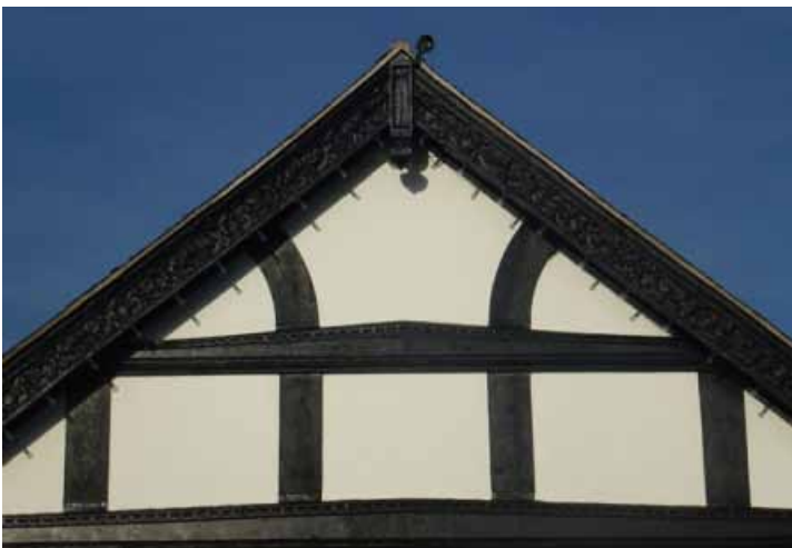
Carved barge boards on the gables © Rory Walsh
