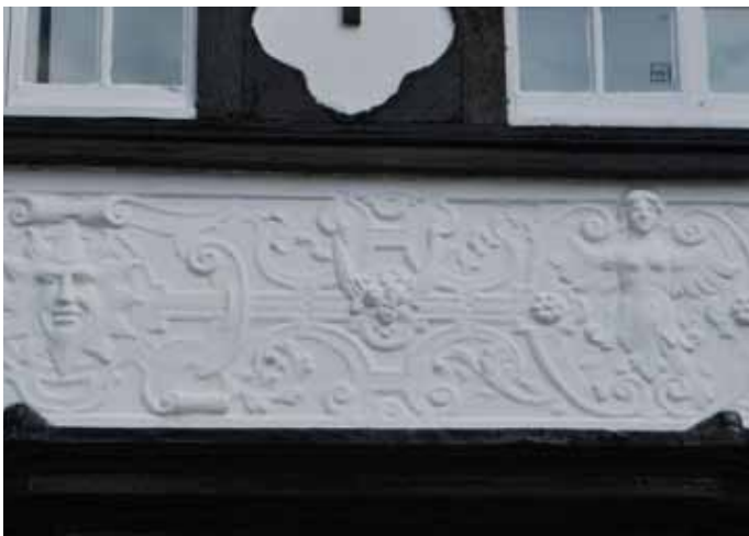
Pargetting above the ground floor © Martin Haslett
